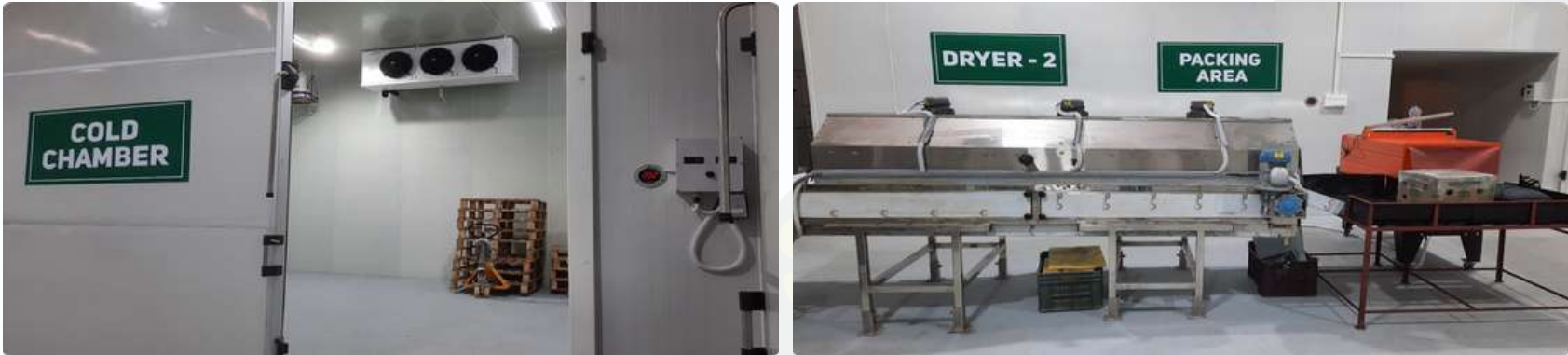
TRIPURA - INTEGRATED PACK HOUSE
